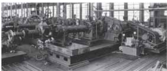
Photo. 2 Single screw extruder - P200(1960)
