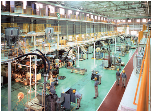
押出実験棟 Extrusion Facilities
