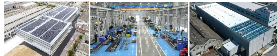
No. 3 Machining Shop, which has commenced operations (left and center) No. 4 Machining Shop, currently under construction (right)
